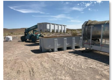
Figure 4: Photo of solvent extraction (SX) equipment being unloaded on site
