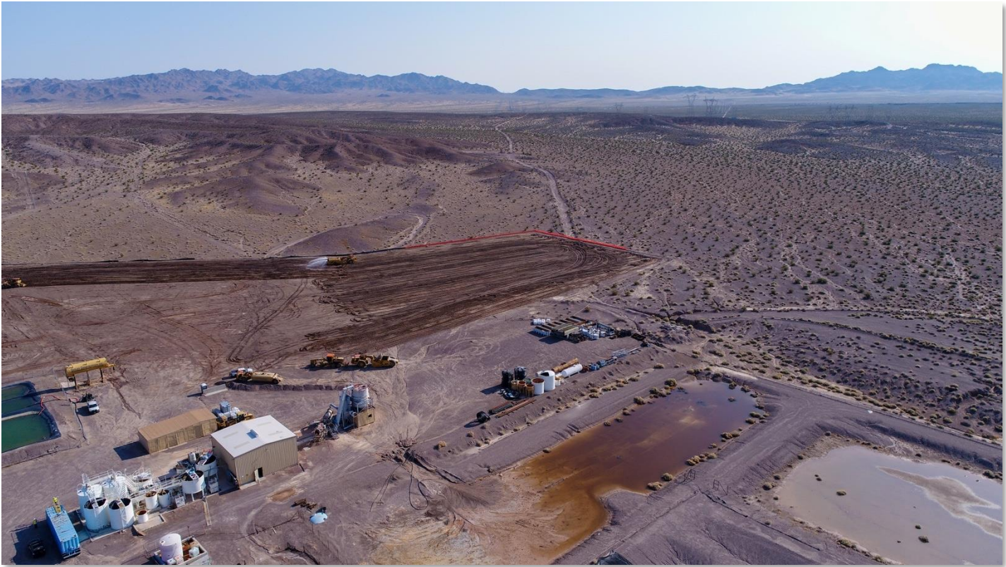
Figure 1: Aerial photo of early site works
