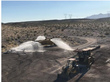
Figure 3: Photo of initial earthwork preparation for plant site
