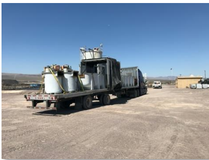
Figure 2: Photo of mixing tanks equipment arriving on site
