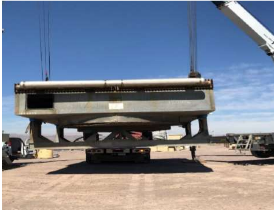
Figure 2: Fin Fan Cooler Delivered to Site
