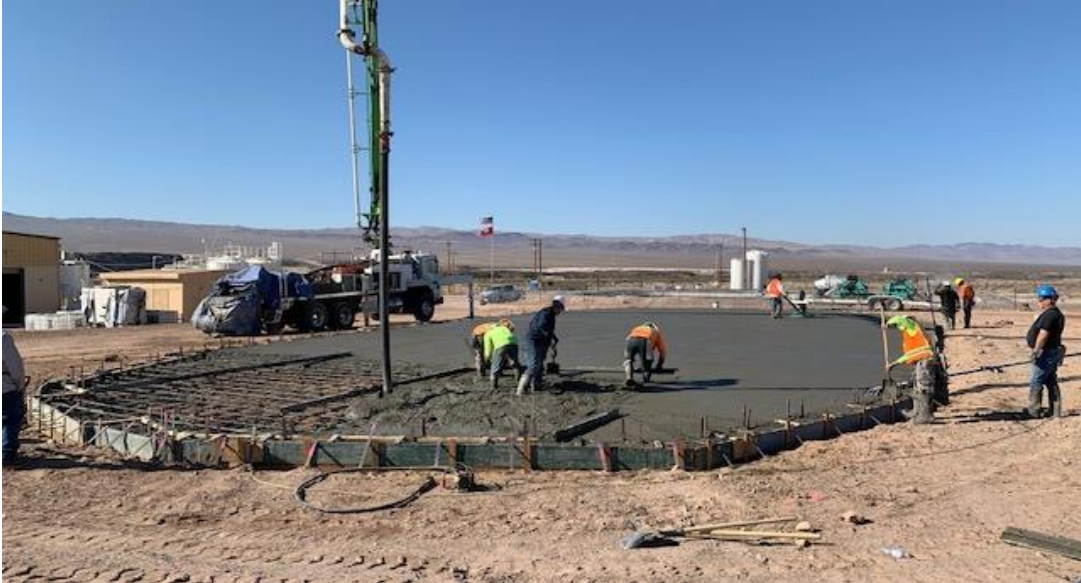
Figure 1: Photo showing concrete pour for materials warehouse
